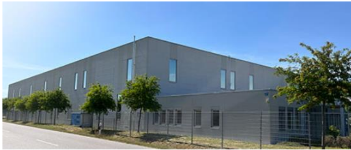
Bausch+Ströbel Werk Sachsen GmbH+Co. KG – projected foundation in 2023 Plant Construction, Engineering, Assembly
